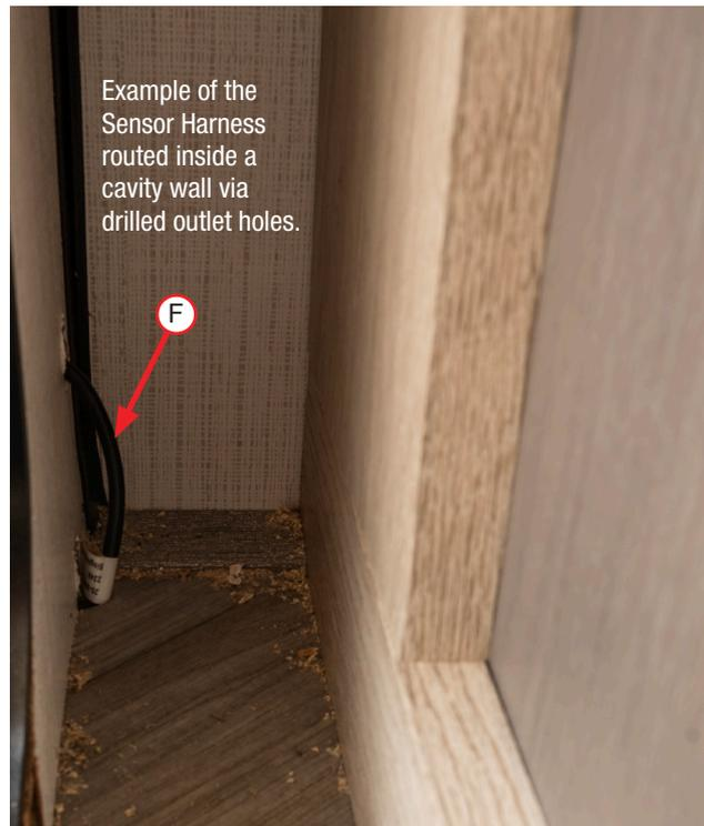
Example of the Sensor Harness routed inside a cavity wall via drilled outlet holes.
