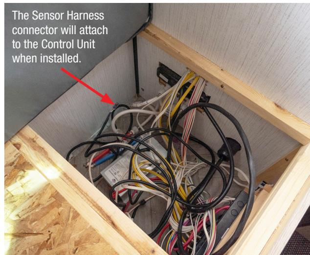
The Sensor Harness connector will attach to the Control Unit when installed.
