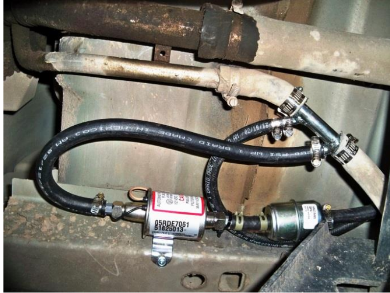
(Fig. 14) Under the vehicle, showing the Vent Line Filler Adapter installed in the vehicle's vent line. Also shown, is the mounted pump, and fuel filter.
