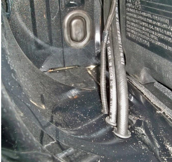
(Fig. 1) Holes for fuel lines and wire loom to pass. Grommets shown installed in fuel line openings.
